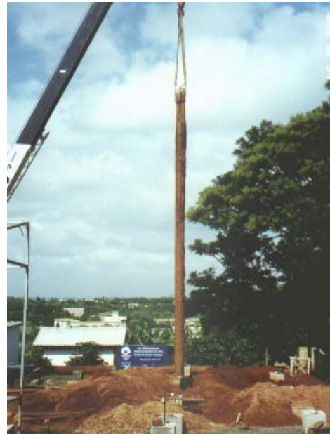
Figure 5. Extracted pile.
